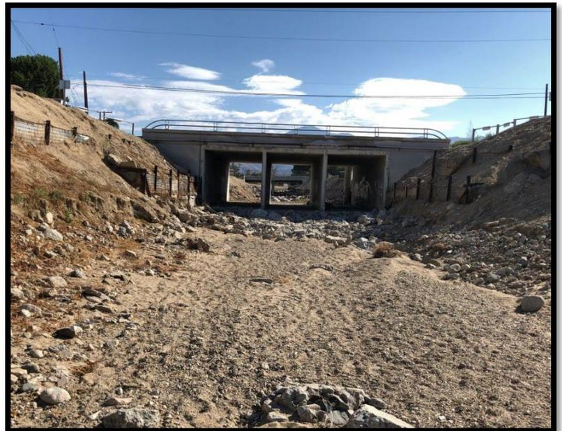
This bridge has several critical functions. First, the structure conveys storm water under Dunlap Boulevard from Wilson Creek which helps mitigate flooding in the surrounding area. Second, the bridge serves as a utility corridor for water, sewer, gas, and telecommunication facilities which serve the local area and the region. Finally, the new bridge will enhance access in the Dunlap area even during major storm events.
