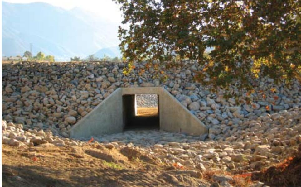
**The 11 by 11 ft (3.4 by 3.4 m) box culvert in basin 3 was designed to return flows to the main channel, helping to reduce high flows and minimize overtopping of levees.**
